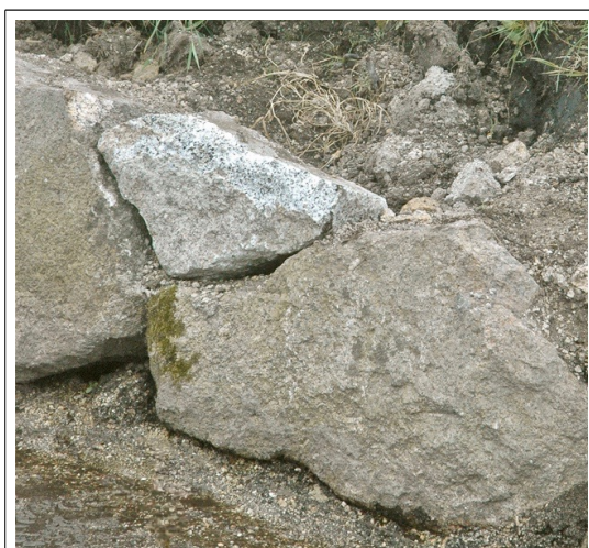
A well-fitting filler stone between two grounders.
