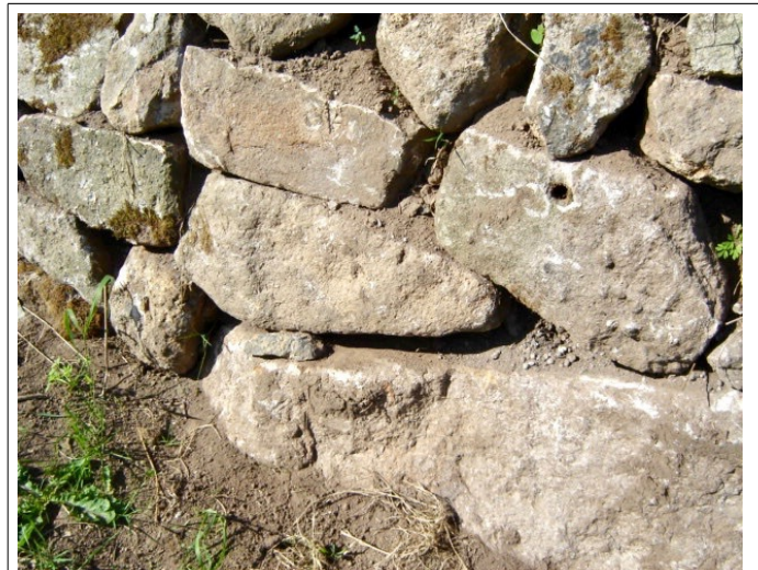
Trig (beneath stone at centre of picture) wrongly used on outside of hedge.
