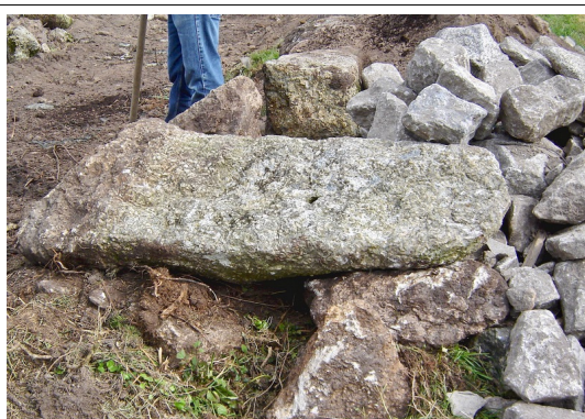
1. Granite gatepost ready to set. Normally about a quarter of the length should be set into the ground. With a lumpy bottom end like this, a little less will do.
