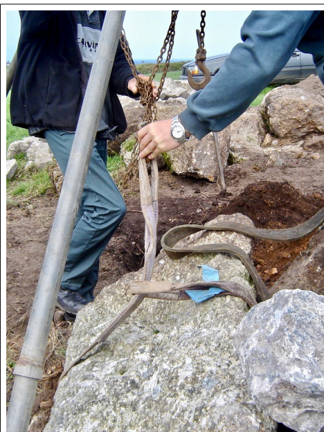
3. The pulley chain is hooked to a strong strap around the gatepost.
