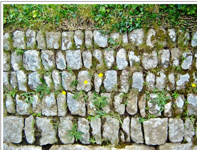
Straight diminishing courses of sorted and partially dressed stone. The varied widths and irregular shapes, while dressed sufficiently to fit well, are particularly attractive at this house frontage. Unusually the grounders are long level slabs of stone - note wider stones across the joints.
