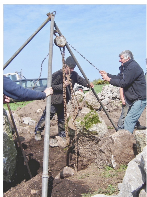
8. Raising the stone just clear of the ground with the endless-chain pulley. Notice that everyone stands clear.
