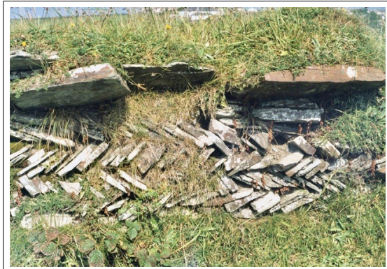
An old slate hedge with large slabs laid in as coping to prevent sheep from climbing over.
