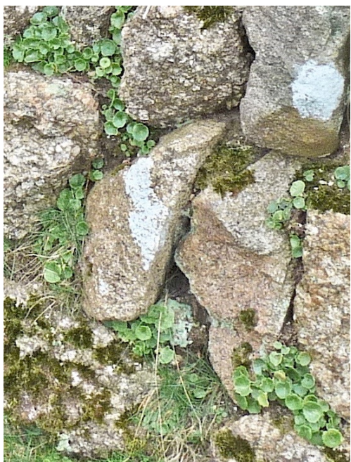
Two "ugly stones" strongly built into an old field hedge in West Penwith. Note good solid well-shaped stones are used around them.
