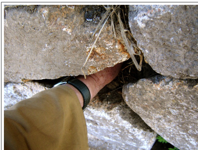
Any gap between stones larger than a tennis ball creates instability and will let rabbits get into the hedge. If it admits a hand, it's too big.
