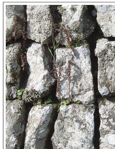
Stones wrongly laid stone above stone with vertical running joints making a weak structure.
