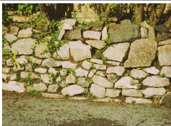
An appallingly badly-built new hedge. Topsoil fill, side bulging out, stone unsorted, big stone above small, higgledy-piggledy placing of stone in the courses, big gaps between stones.
