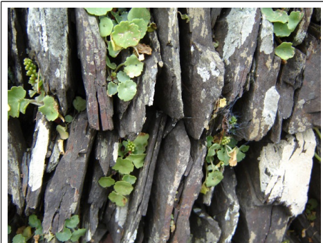
Slate 'pitchers' or 'edgers' must be fitted stone-to-notch between courses.
