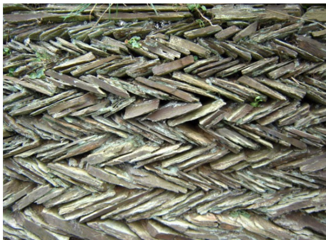
'Jack-and-Jill' herringbone slate hedge. Some errors in laying. Angling the slates a little more steeply and regularly would have improved stone-to-notch interlocking and made slates less likely to slide outwards.
