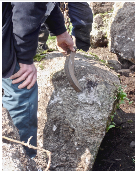
5. Hooks placed in the notches ready to grip.
