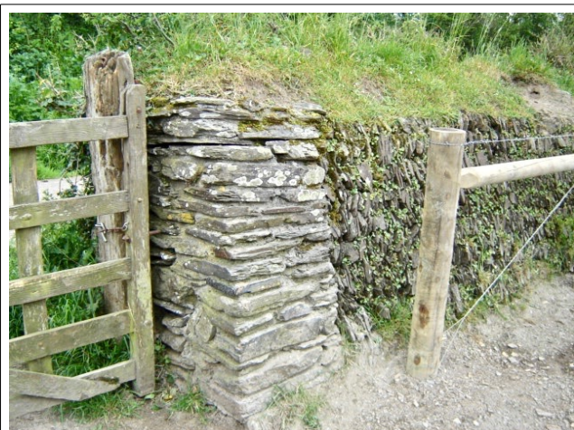
Hedge-end in slate country built with lime mortar to stabilise gateway opening and make a firm housing for gate fastenings.
