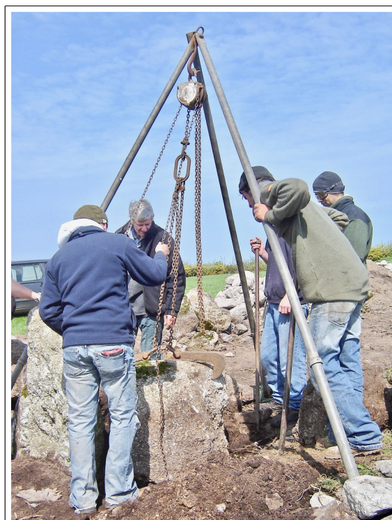
9. The stone has swung into the centre of the tripod and is lowered to the ground, ready to unhook, move the tripod forward and repeat the process until the stone is in its final position.
