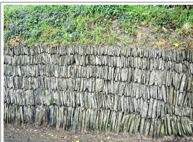
Pitched slate. Note good interlocking courses, no earth or turf between.
