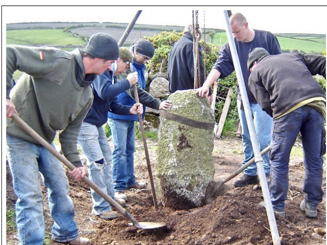
7. The hole is filled in and the soil well rammed.
