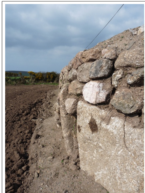
Poor use of large facer in foreground set upright with another beyond and alongside it which is moving outward at the top, so stones above will fall down.
