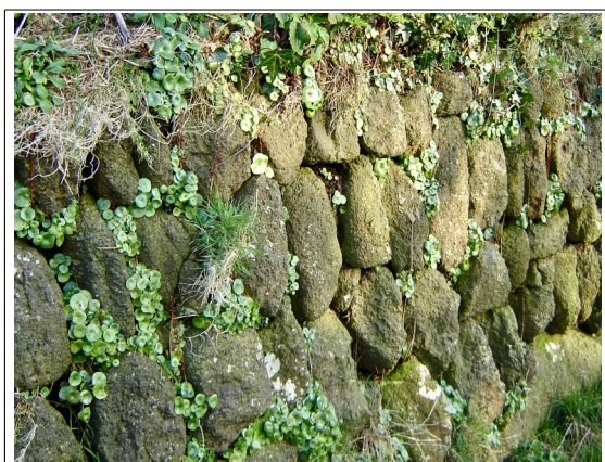
The beauty of this typical old country-built West Penwith hedge lies in the weathered shapes of the granite moorstone smuggled together by the hedger's skill.
