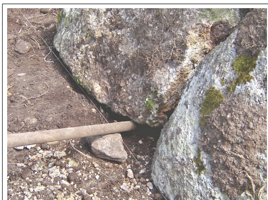
Using a stone as a fulcrum to rest the bar on while levering up a large stone to adjust its position. Note, the shadow makes this look like a triangular stone, but of course it is not. The shape must be stable to rest on or the bar will move or slip off.
