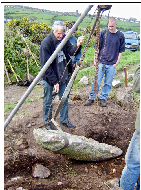
5. The strop has been moved higher up the post for the pulley to raise it.
