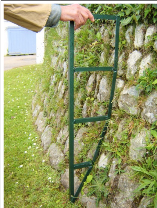
This well-built 4ft hedge has already kept its batter for nearly a century and has never lost a stone in that time.
