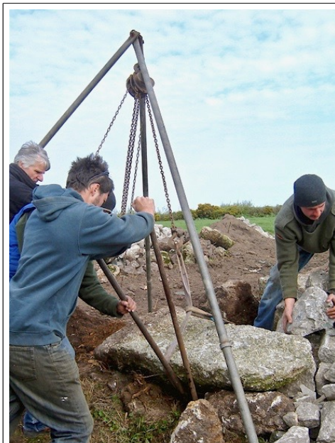
4. The chain block takes the weight as the gatepost is guided into position with long bars.
