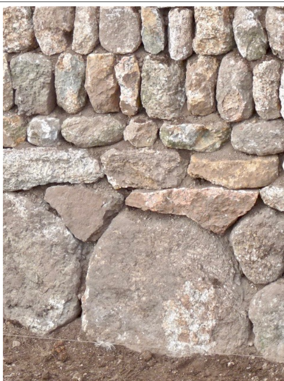
Courses from bottom up: grounders, fillers, two rows laid flat, two rows pitched.
