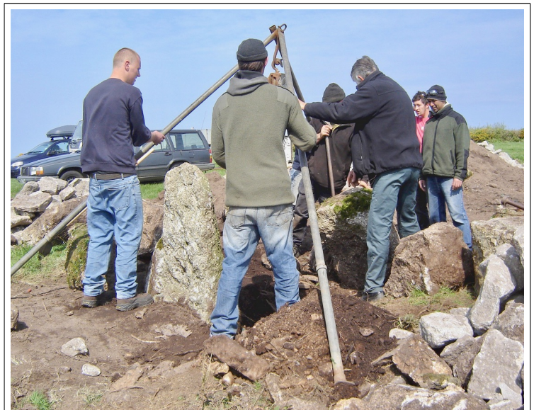
3. The tripod is positioned with centre a little ahead of the stone, which can be seen between the near tripod pole and the instructor's left leg.
