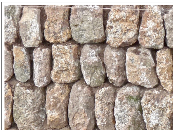
Three rows of pitched granite, with well-broken joints.
