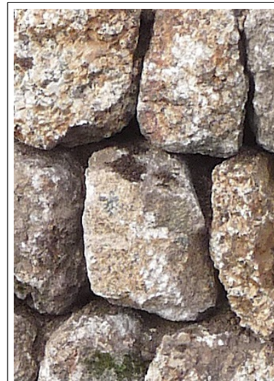
Stones correctly laid with broken joints, stone above join, making a strong hedge.
