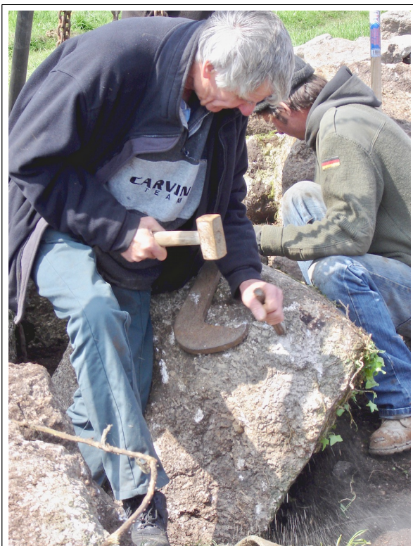
4. A notch is made in the stone each side to give a grip for the hooks.
