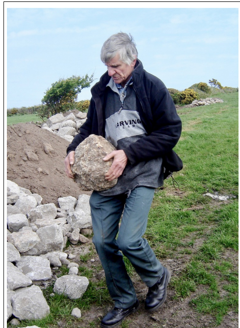
Carrying a stone supported against the hip and thigh. Note back is straight and knees slightly bent.
