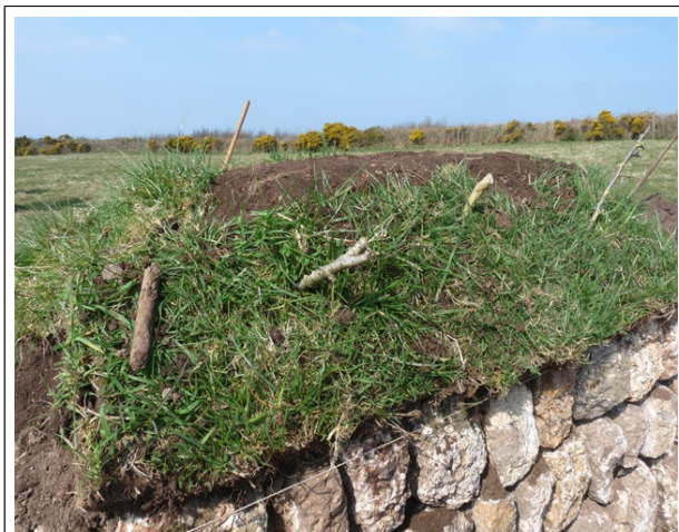
Tobs are laid on the domed top of the hedge and pegged down.
