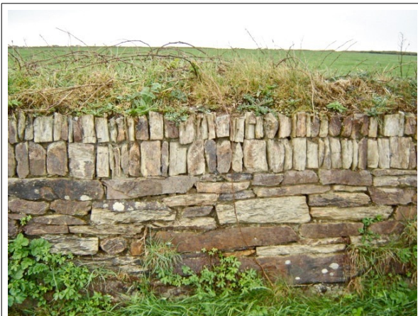
Unusually well-built recent hedge of shale laid on the flat (horizontally). The top two courses of stone are pitched ('edgers') to make a strong hedge top.
