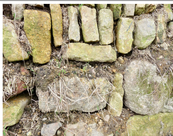
If earth fill is wrongly placed between the courses like this the stones will move outward, causing collapse.
