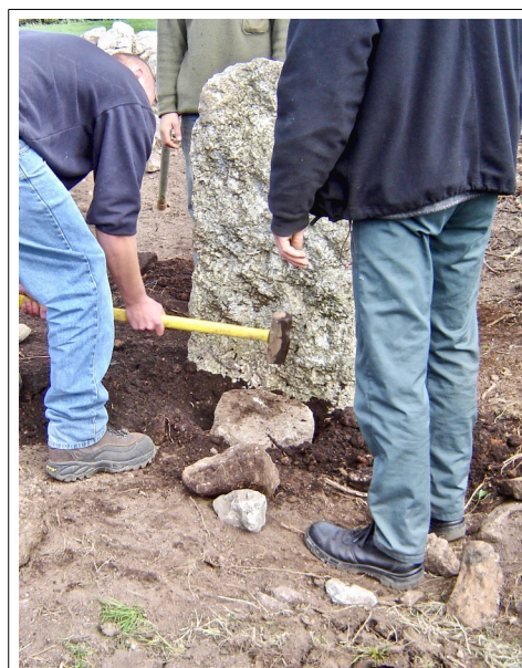
8. A flat-topped stone is set in at ground level on the gate side of the post.
