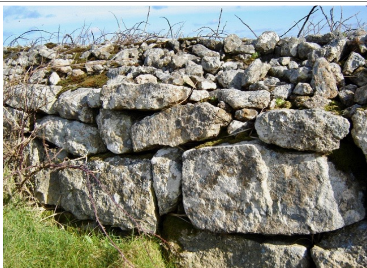
Stone hedge with small field-picked stones used as fill and capping. The capping on this type of hedge is sometimes of rab or of peat.
