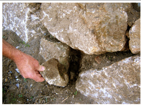
If any stone (excepting in the top row) can be removed by hand, it has not been properly built into the hedge.
