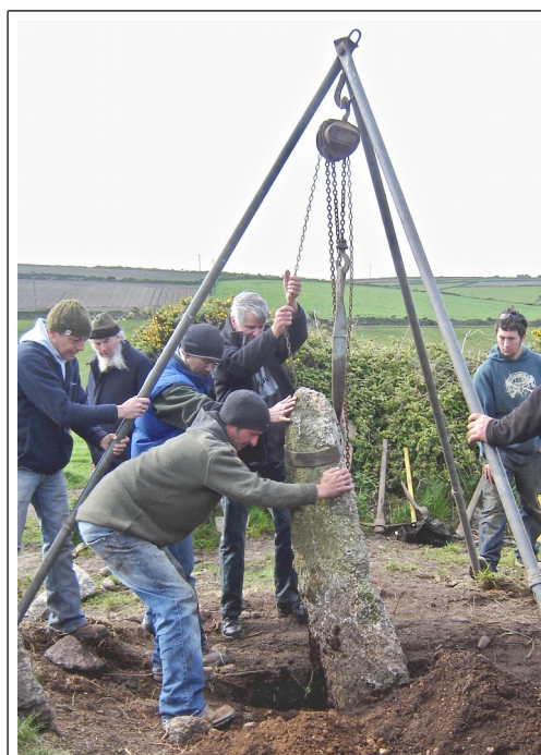
6. The gatepost is straightened as it settles into the hole.
