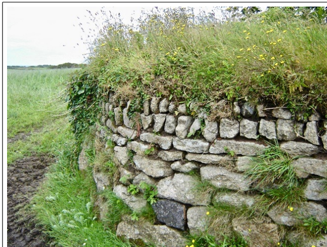
Hedge end rounded off into gateway. The hedger has made a neat job but has lost the curved batter.
