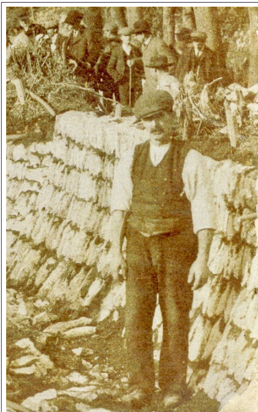
Rare photograph of the winner at a Cornish hedging competition around the end of the 19th century shows the hedge built to the traditional batter curve. The hedger's shadow shows the curve exactly fitting the batter recommended by recent champion hedgers.
