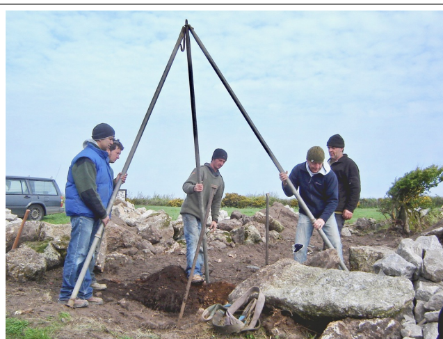
2. The tripod is positioned over the hole dug to receive the gatepost.
