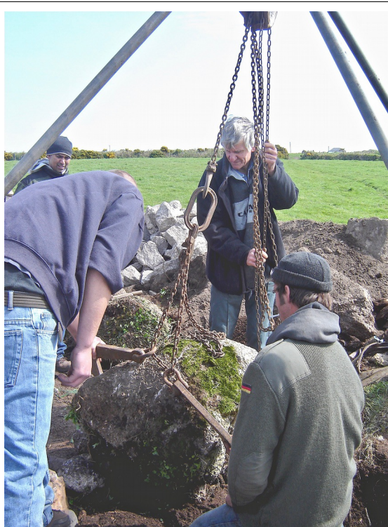
6. Taking up the slack on the chains.
