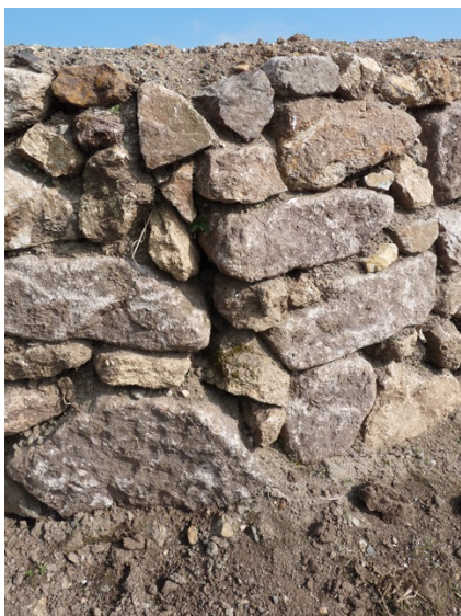
A bad running joint already opening up in this very poorly-built new hedge. Another running joint at right of picture means the whole section between them is already bulging and is going to fall out soon.
