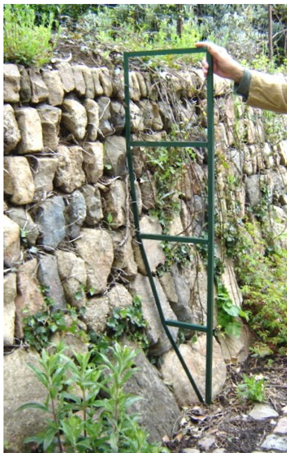
Correct batter on a 5ft retaining hedge over 100 years old. Recent removal of green cover not a good idea but shows the stonework still in perfect condition.
