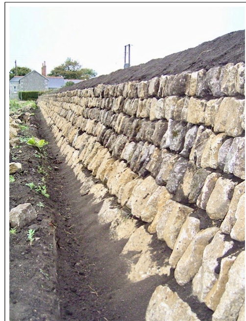
A new Cornish hedge at Ashton built without using a line. Photo: Mark Kelmanson
