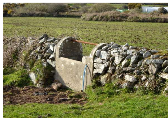
A neat little concrete drinking trough not so neatly set into a hedge.
