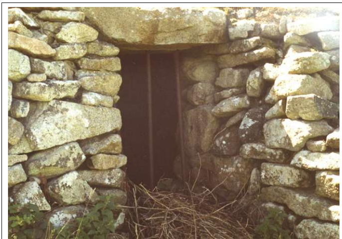
Pig's creep built into a stone hedge. (The bars have been added since the creep was disused, to dissuade people from entering.)
