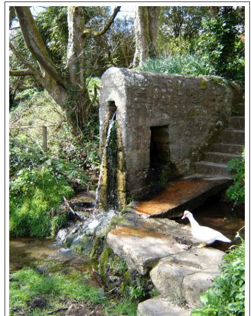
A spout built in the higher hedgebank catches the water of a spring running into the main stream. The square opening in the side was built to put a cloam pitcher in to fill under the internal pipe, giving a controlled supply even in times of heavy rain when the overflow, seen running in the picture, is gushing too fast for easy filling
