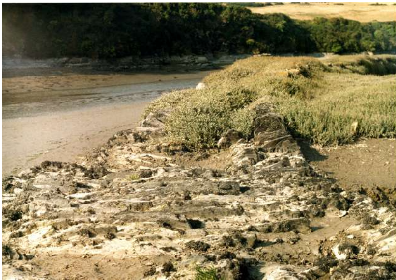
Slate-built Cornish hedge enclosing pool for tide-mill on the river Camel. Foreground section breached by the sea shows basic construction.
