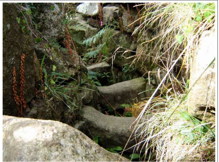
Coffen stile in a former deer-park built with a curve through the hedge to prevent deer from jumping across.
