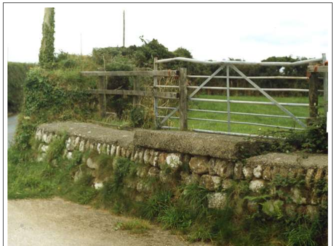
Churn stand built on adapted section of Cornish hedge which could still be used to off-load fertiliser etc into the field.
