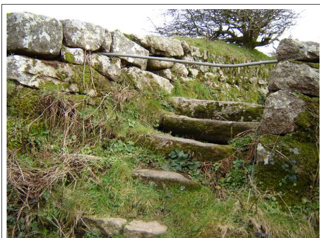
Picturesque, traditional stone stile is in character with local landscape and geology, safe and easy to climb, and will last for centuries with minimal maintenance.
