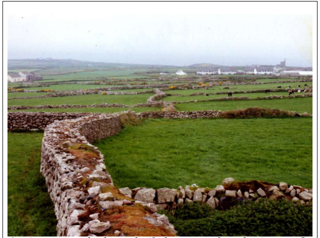
Ancient stone hedge rebuilt by unemployed miners. In rebuilding, the kinks typical of prehistoric hedges showing where other hedges have been removed, to enlarge the originally tiny fields, were smoothed out into curves.
