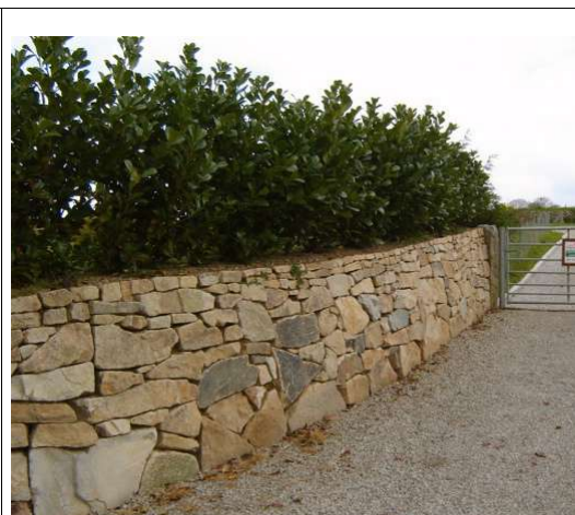
With the best of intentions, work directed towards tourism can alter the landscape that people come to see. While Cornish hedges have been built at this new entrance, their style and chosen planting is not traditional and the end result looks suburban and out of character.
