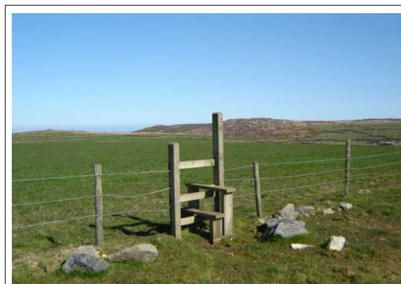
Wire fence and wooden stile are out of place in Cornwall. They mar the character of the landscape, posts soon rot and stiles become slimy in the Cornish climate, dangerous and difficult for the less-able to climb. Fences allow run-off erosion on the rain-lashed sloping land, whereas a good Cornish hedge prevents flooding downhill.
