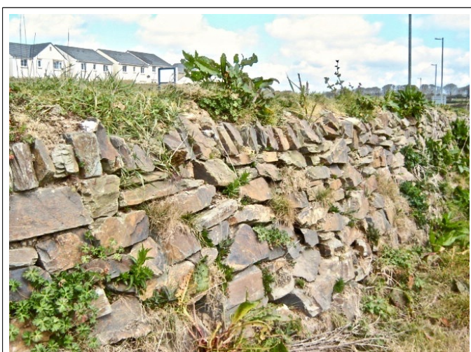
Unfortunately now typical poorly-constructed contract hedges built of cheap shale in higgledy-piggledy so-called 'random coursing', with topsoil fill. Poor specification and lack of skill result in problem hedges with frequent and sometimes spectacular collapse.
