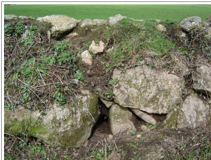
Typical rabbit entry in an old, poorly built hedge, as found on some 19th century miners' smallholdings.
