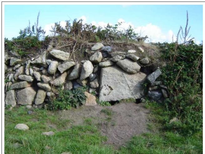
Hedge carelessly built on the surface of the ground instead of setting the grounders in to a proper depth allows rabbits to enter at ground level.
