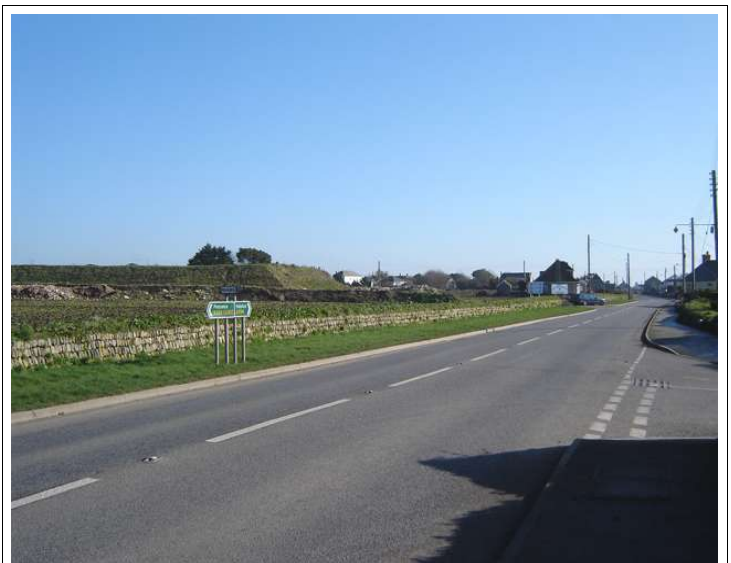
New Cornish hedge (built 2004) alongside the Penzance - Helston turnpike, now the A394.
