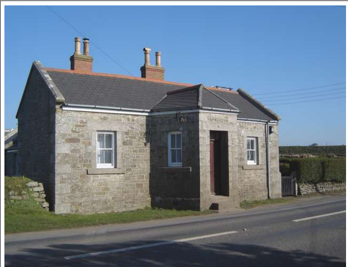
Toll-house, dated 1804, on the Penzance to Helston turnpike road. The toll-keeper sat inside the projecting booth with a window to each direction.
