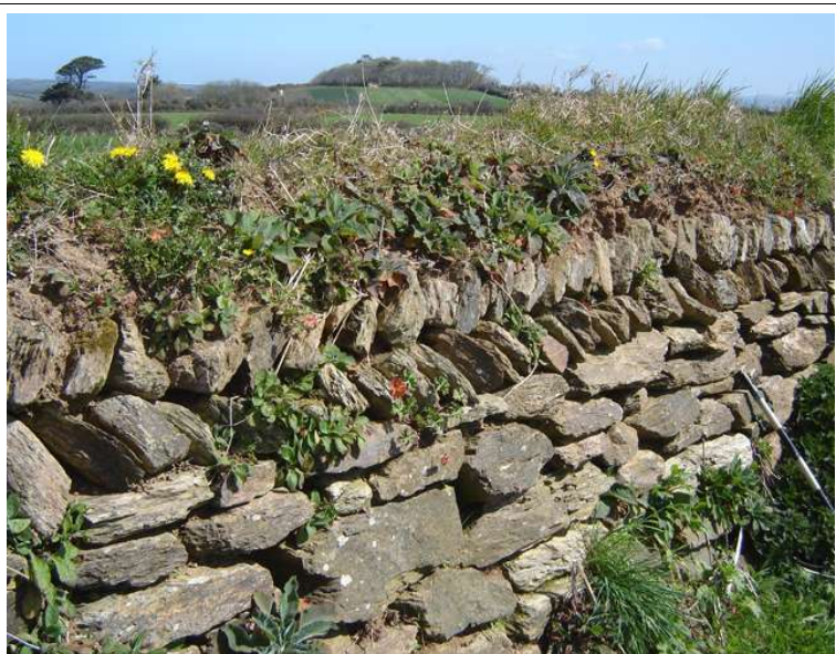
Typical recent roadside hedge of shale, often inappropriate to the local geology as is the case where this one was built near Penzance.
