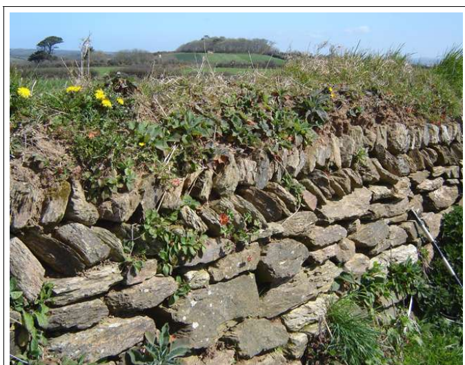
Typical recent roadside hedge of shale, often inappropriate to the local geology and hedging style as is this one built near Penzance.
