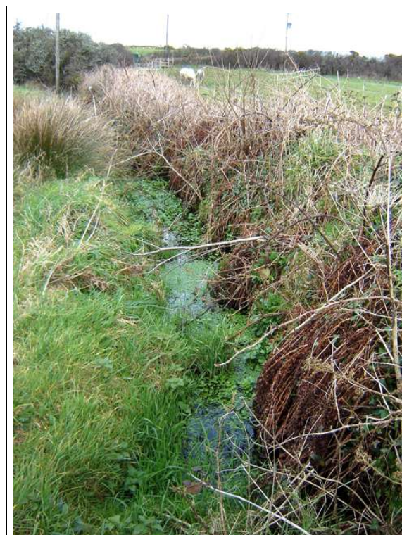
Ditch and verge lying between road and hedge may complicate land-owning issues.
