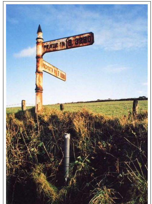
Hedge-top cast-iron signpost looks picturesque and is easily visible. Unlike the ugly modern sign already broken and gone from here, the old signs will last for centuries with only a coat of paint now and again - which this one near Black Rock urgently needs. Many of these fine historic signs are today suffering this kind of disgraceful neglect.
