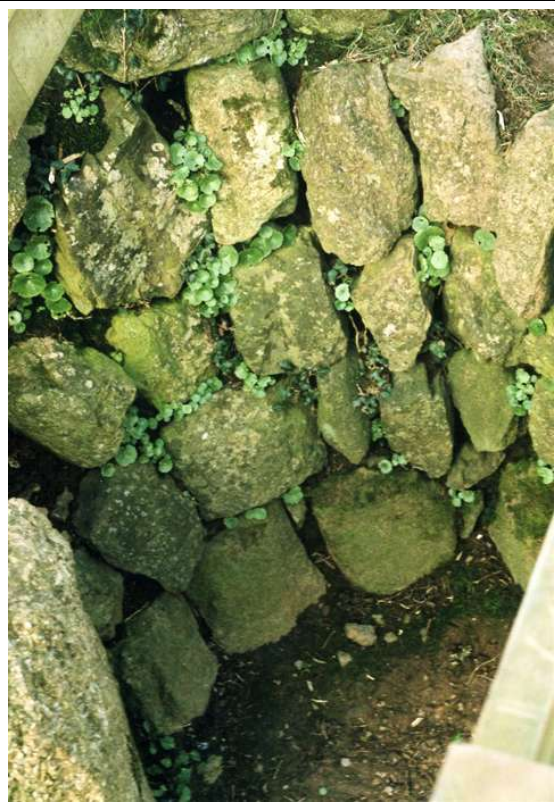
Looking down into the gap showing the batter built into the curved hedge containing the kissing-gate.
