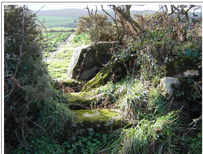
While this is easy for walkers, it is a shame to see stiles like this fall into disrepair with the current decline of stock-farming. The top tread of this fine old cattle stile has fallen (seen on right, slanting down) but could easily be replaced in position.
