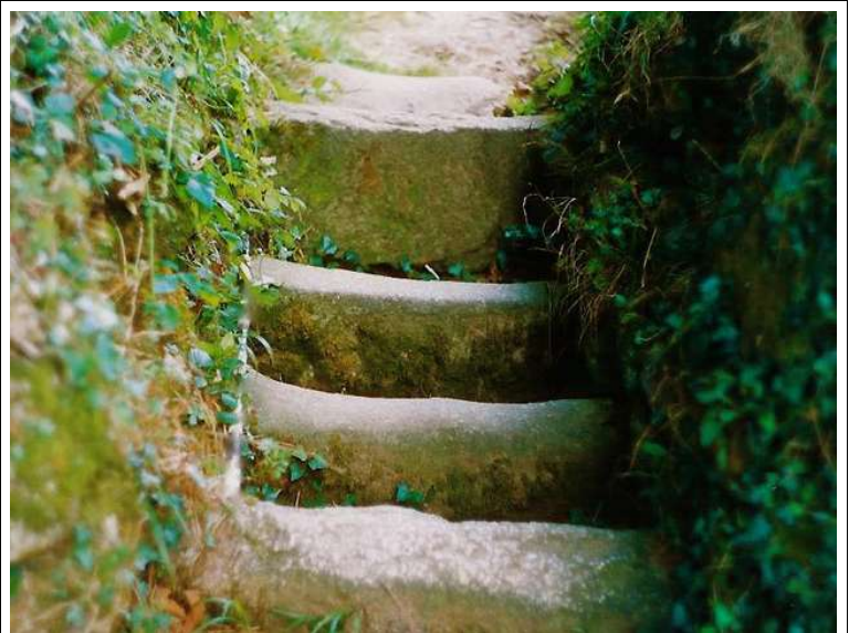
Coffen stile with four level treads.
