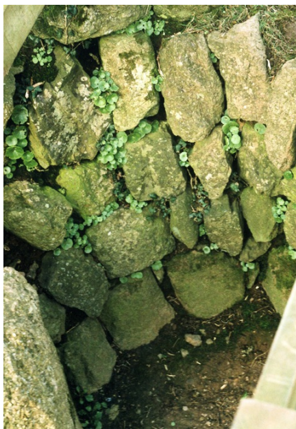
Looking down into the gap showing the batter built into the curved hedge containing the kissing-gate. Built in traditional style with undressed stone fitted together.
