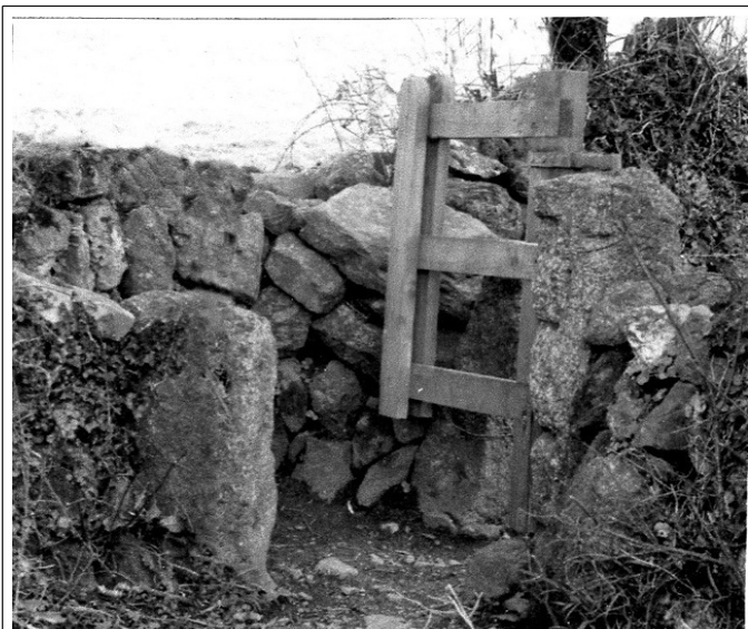
Unobtrusive kissing-gate built into a Cornish hedge in a traditional style using local stone. An iron gate would suit the climate and the traditional Cornish ambience much better.
