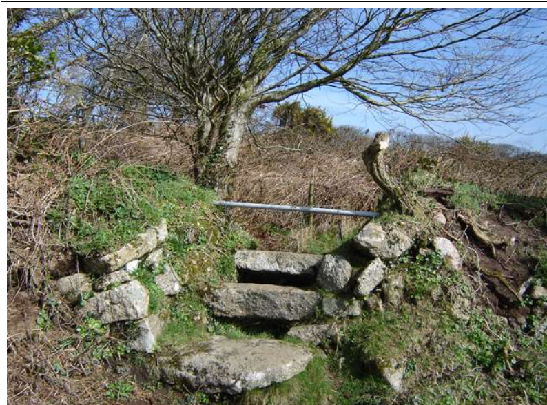
2" galvanised water pipe set in above cattle stile to keep livestock in, forming easy step-over function.
