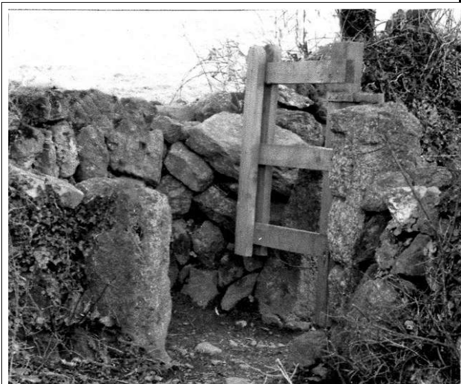
Unobtrusive kissing-gate built into a Cornish hedge in a traditional style using local stone.
