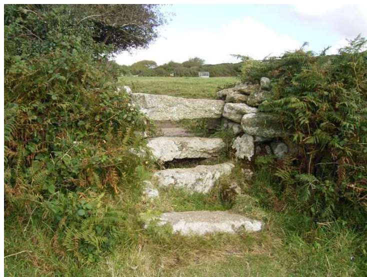
This cattle stile of three treads and a foot-stone has been raised by adding another stone tread at the top of the hedge to keep modern livestock in.
