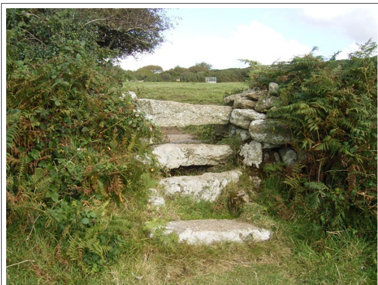
This cattle stile originally of three treads and a foot-stone has been raised by adding another stone tread at the top of the hedge against modern livestock.
