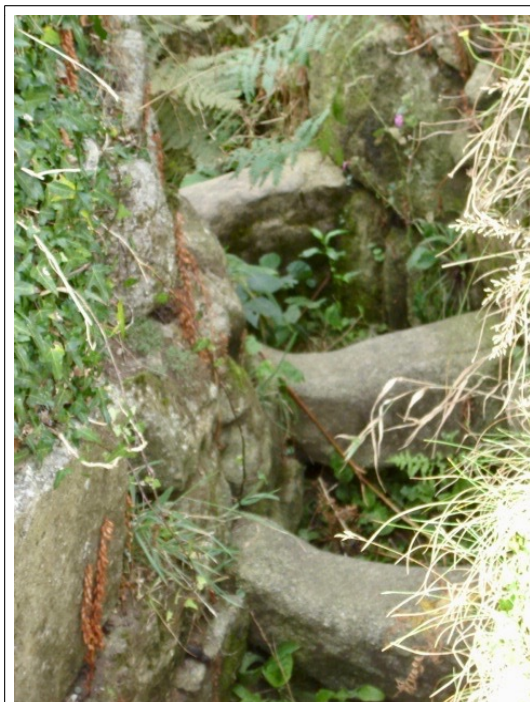
Coffin stile built with a curve to keep deer in. Worn treads show great antiquity.
