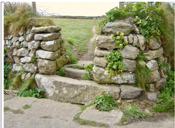
This coffin stile unusually has a step up on one side to allow for a drop in ground level.
